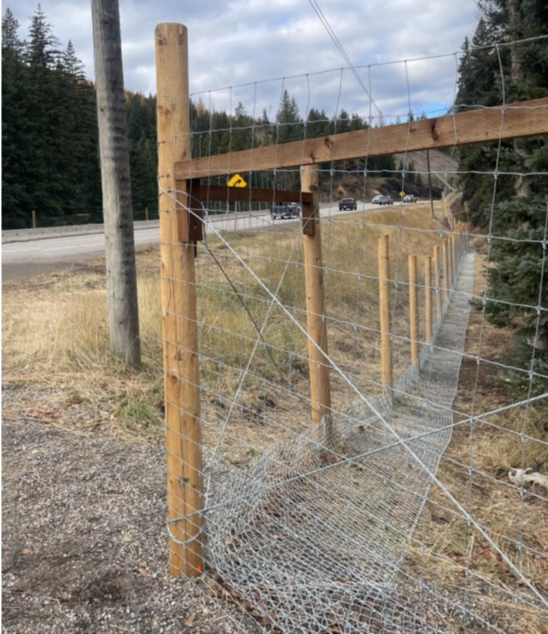
*Image 7. Phase two wildlife exclusion fencing between Carbon Bridge and Alexander Bridge. Chain link skirting to reduce animals digging under the fence shown at the bottom.*
