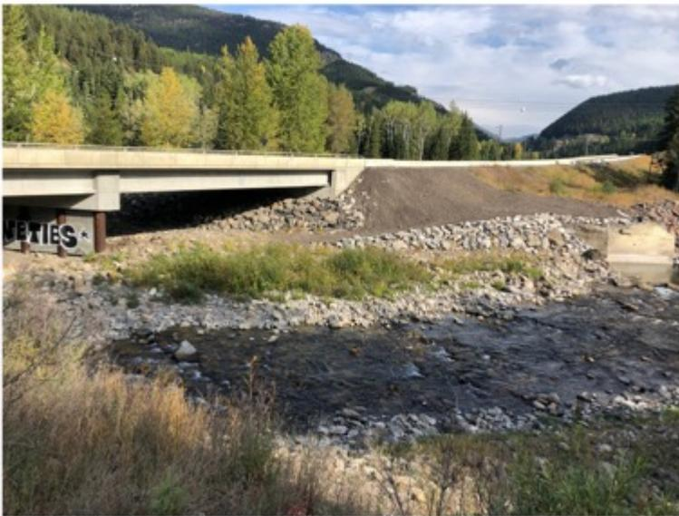
*Image 2. Example of an underpass retrofit at Loop Bridge. Here a large open span bridge had the potential to provide an effective underpass below the highway, but rip rap and an old abutment blocked animals from easily entering the river edge. We removed a portion of this abutment and created a 10 ft wide path down to the underpass that makes the structure more enticing and safer for wildlife.*
