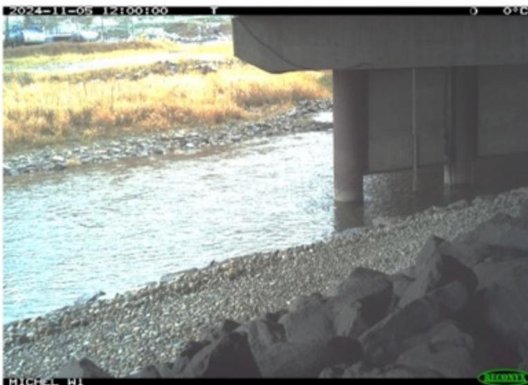
Image 4. Example of an underpass retrofit at Michel Mouth Bridge. A similar approach to Alexander Creek was used here, where a 1.5 m wide path was created through the large rip rap and filled with pea gravel to create a surface more ammenable to wildlife use on both sides of the bridge.
