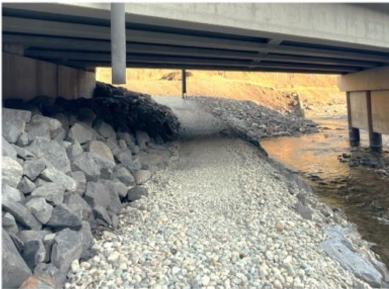
*Image 5. Example of an underpass retrofit at Old Town. A similar approach to Alexander Creek was used on the NW side of the bridge, where a 1.5 m wide path was created through the large rip rap and filled with pea gravel to create a surface more amenable to wildlife. The SE side of the bridge was already very open and serving as an underpass with no work needed. use.*
