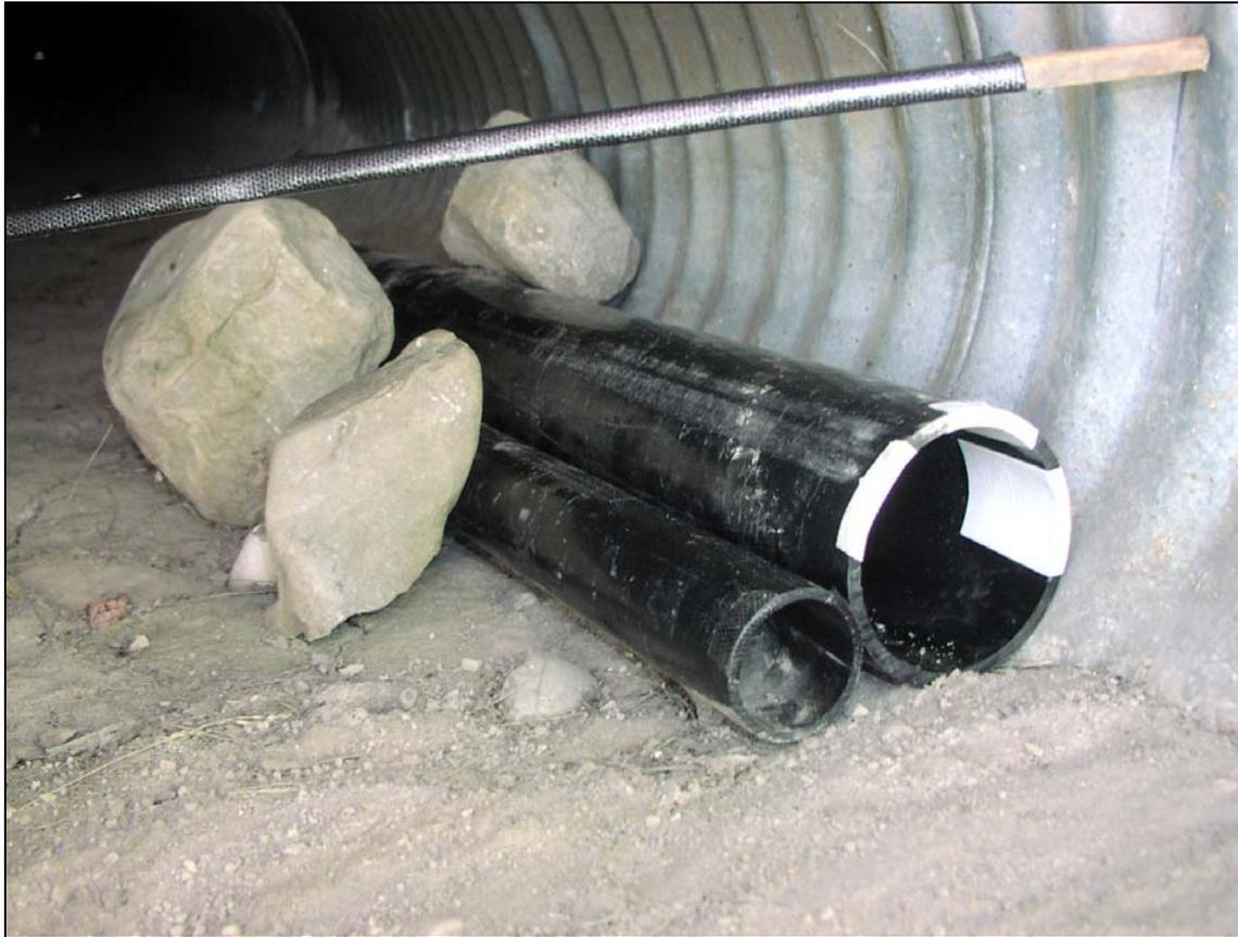
*Pipes placed in culverts to provide cover for small mammal movement (Photo: Tony Clevenger).*
